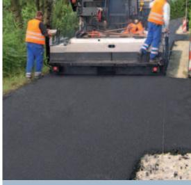
Variomatic screeds - ideal for flexible paving widths.
