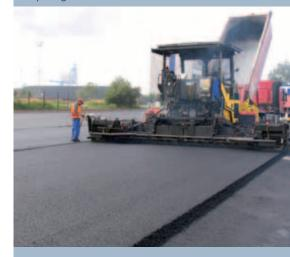
· Fixed screeds for large width paving.
