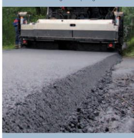
Paving thicknesses up to 300 mm.
